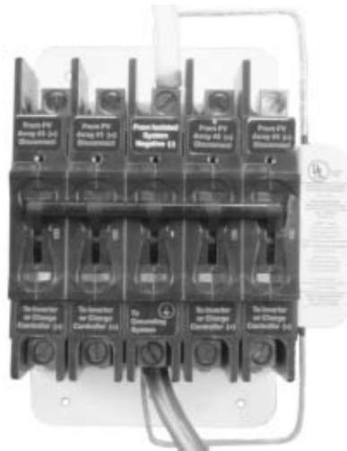
Figure 2-16 PV Ground Fault Protection (PVGFP)
