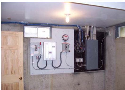
Painted plywood board in basement (BPVS)
