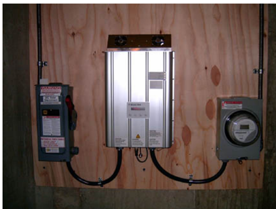
Typical mounting on plywood board (Sunlight Solar)
